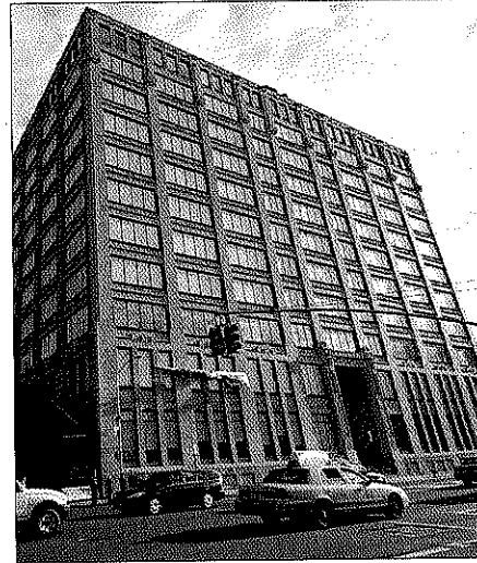
Jones Lang LaSalle is undertaking a gut renovation of the Ogilvy Building at 636 11th Avenue.
